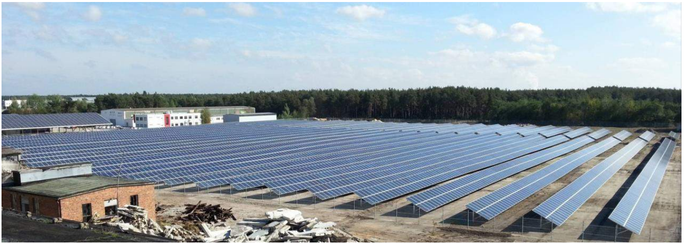
5.3MW Ground-mounted PV Plant in Arneburg, Germany
