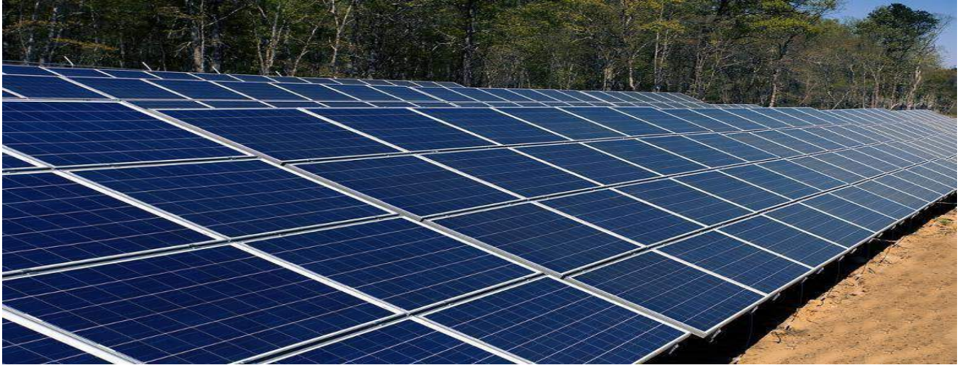
12.8MW Ground-mounted PV Plant in Melksham, UK
