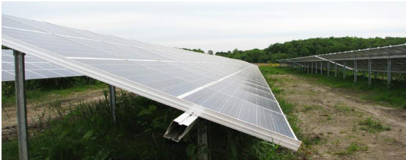
2MW Ground-mounted PV Plant in Guntramsdorf, Austria
