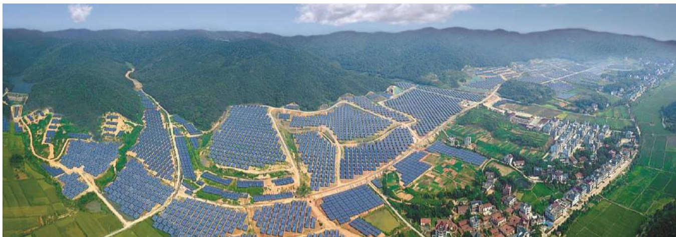
6MW Ground-mounted PV Plant in Exmouth, UK
