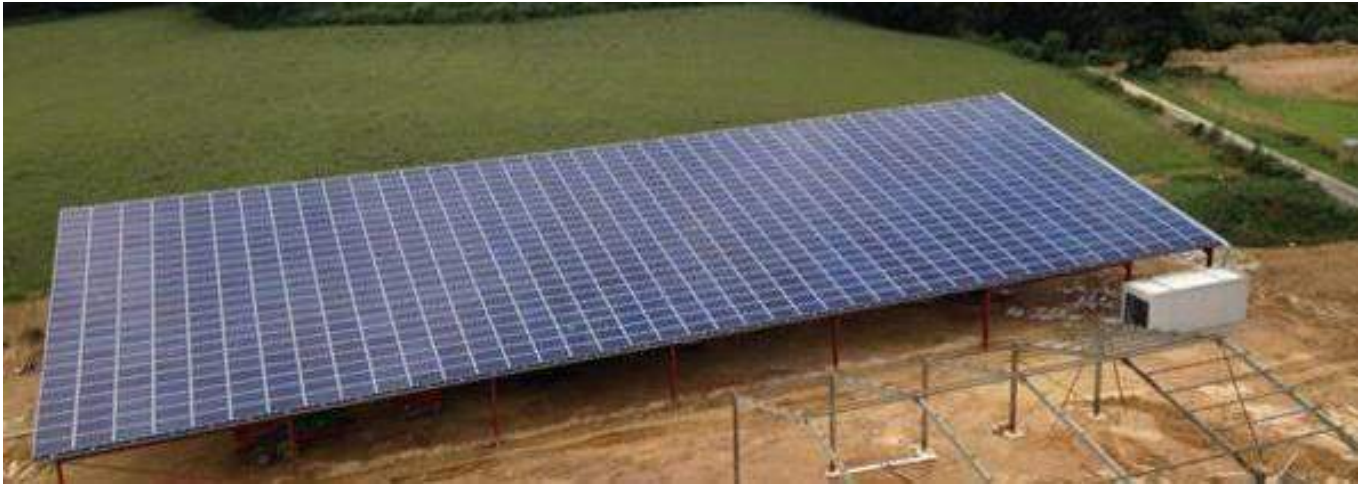
1.7MW Ground-mounted PV Plant in Friedland, Germany
