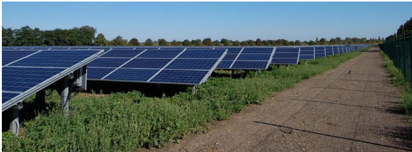
6.3MW Ground-mounted PV Plant in Rooksbridge, UK
